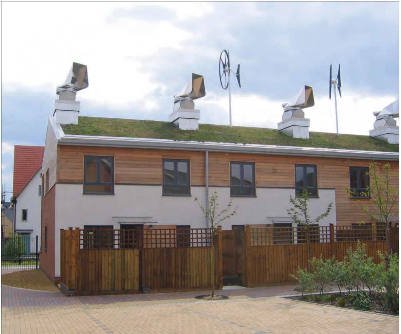
Figure 2 Green roofs on houses in the Upton Development, Northampton, UK.
