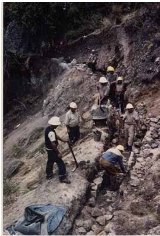
▲ Rebuilding an irrigation canal © Cusichaca Trust
