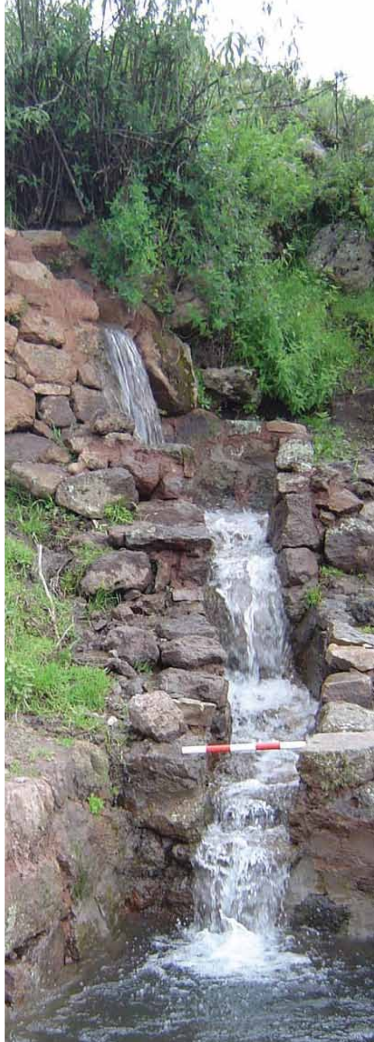
Rehabilitated irrigation canal © Cusichaca Trust
