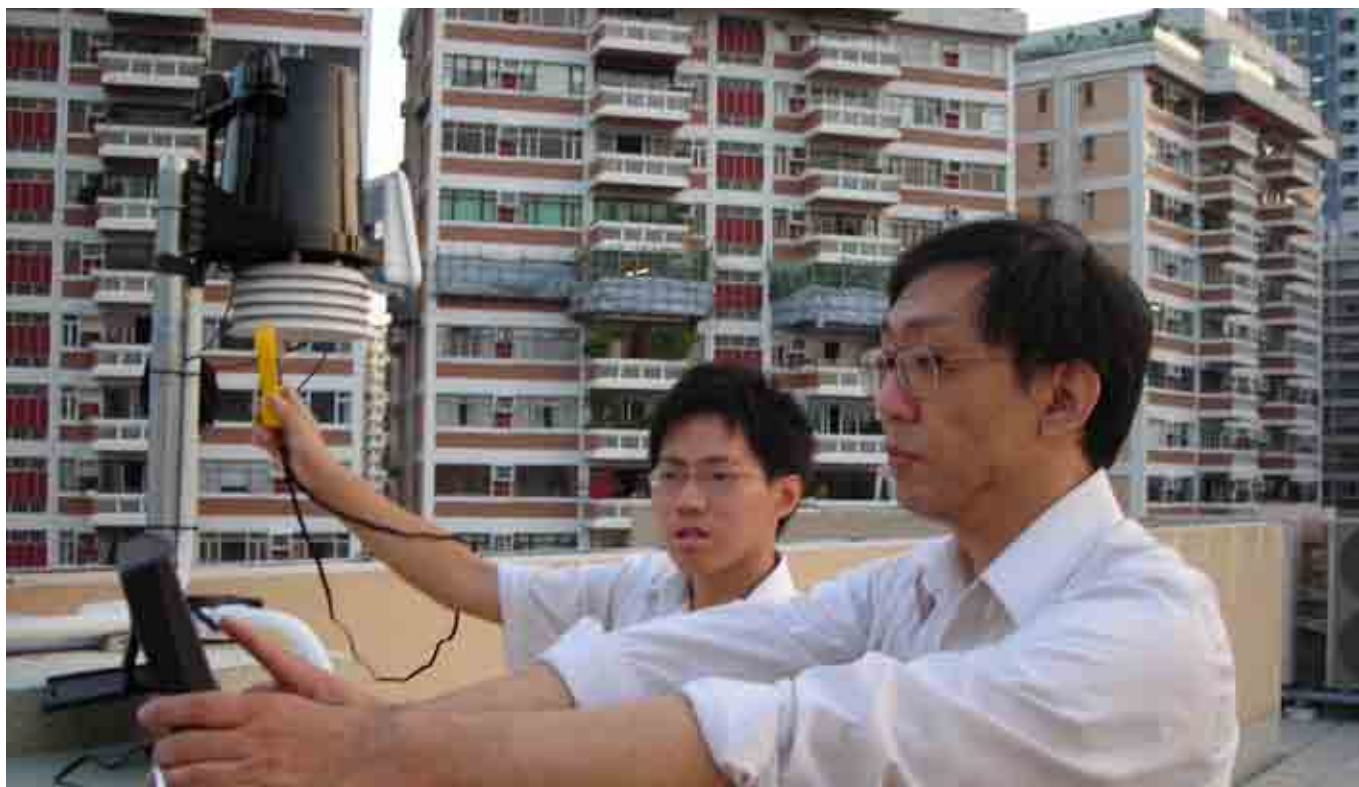
▲ Figure 1. Installing an automatic weather station (AWS) on the rooftop of a school, including a temperature sensor, a humidity sensor, a rain gauge, solar and ultraviolet radiation sensors, and a small display console.
