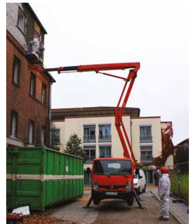
▲ Figure 6. Selective deconstruction (windows, asbestos, etc) of a school prior to demolition. (© Thorsten Kallnischkies)
