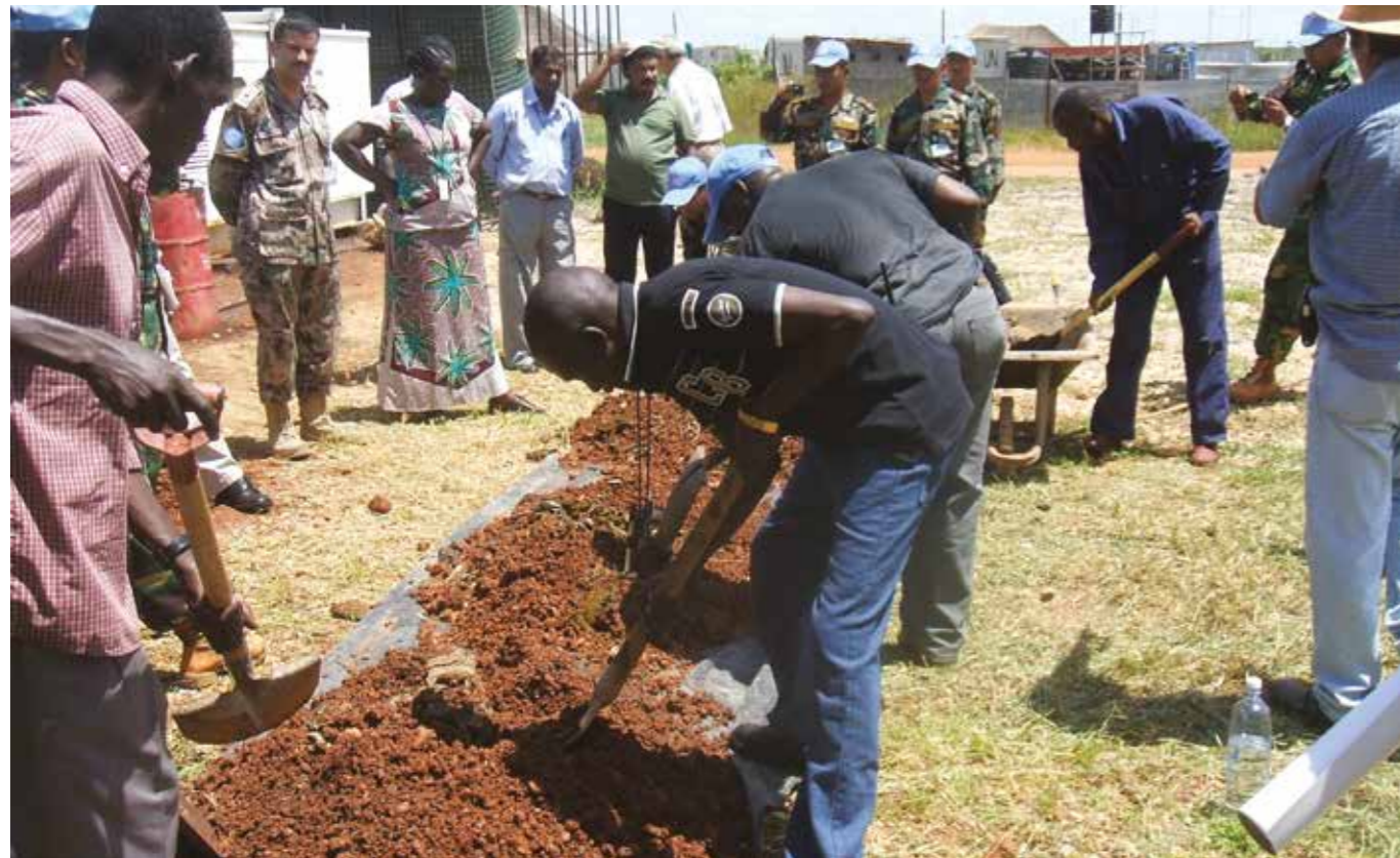
▲ Figure 3. Remediation of an oil spill using easily available local materials. (© Swedish Defence Research Agency)
