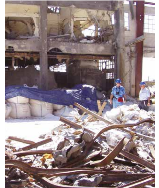
▲ Figure 5. Bomb damage to a glass factory in Lebanon in 2006, which exposed several dozen tonnes of soda ash. This constituted a hazard to cleanup workers and the neighbourhood. (© Thorsten Kallnischkies)
