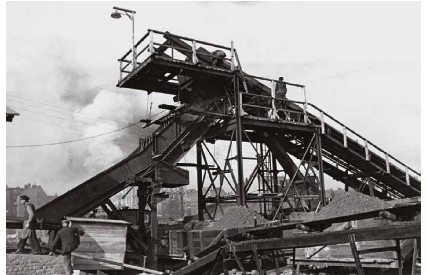
▲ Figure 3. Rubble classifier in Hamburg (1948), which processed 200 t/h. (© SZ Photo/Süddeutsche Zeitung Photo)
