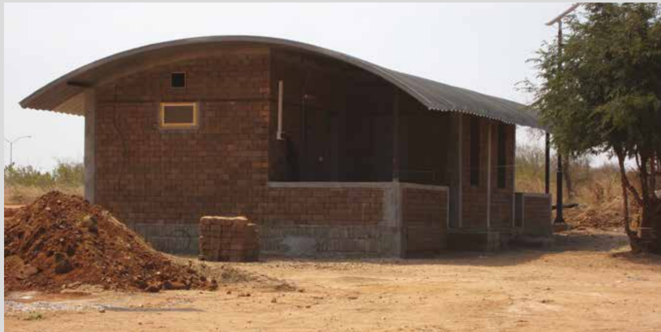
▲ Top: the pilot containers had solar panels and insulation added for use as living/office space or for ablutions. The picture shows (left to right): a control unit (with no solar panels or insulation), an ablution container and a living container (that could also be used as an office).
