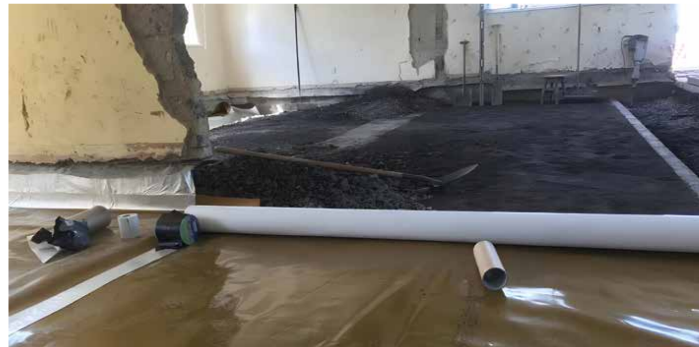
▲ Figure 9. Vapour membrane installed under the concrete subfloor. (© Avada Environmental Ltd)
