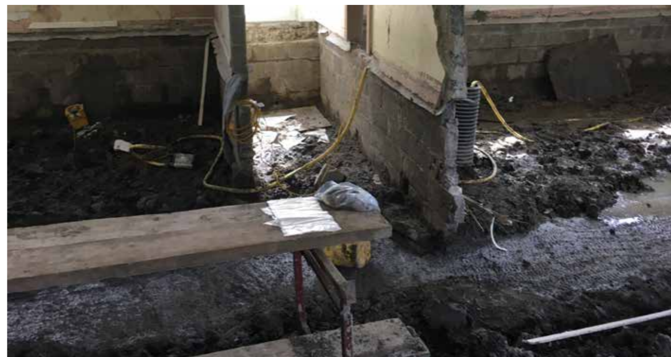
▲ Figure 5. Internal excavations. (© Avada Environmental Ltd)
