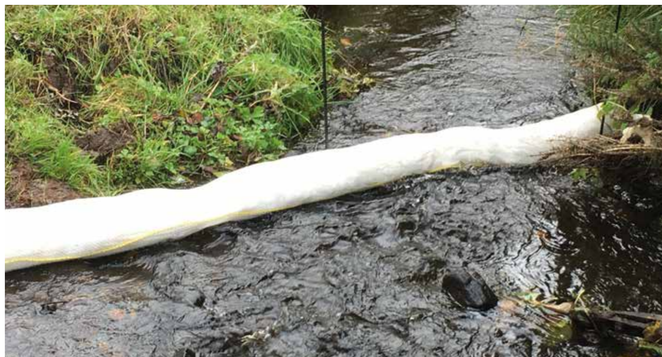
▲ Figure 4. Oil boom installed at the nearby river. (© Avada Environmental Ltd)
