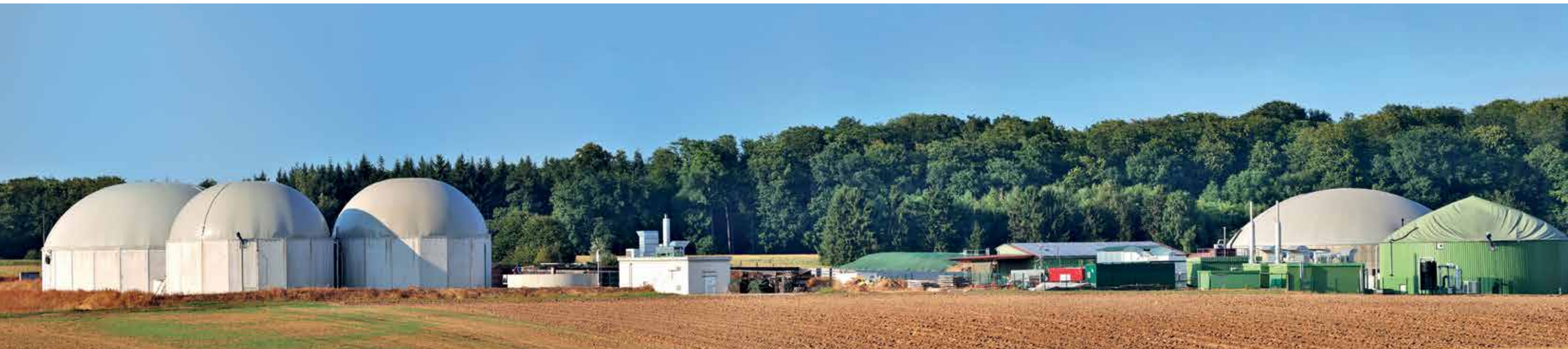
▲ Figure 2. An anaerobic digestion (AD) facility, which can recycle food waste to generate biogas which can be used to produce renewable energy. (© loraks | Fotolia)
