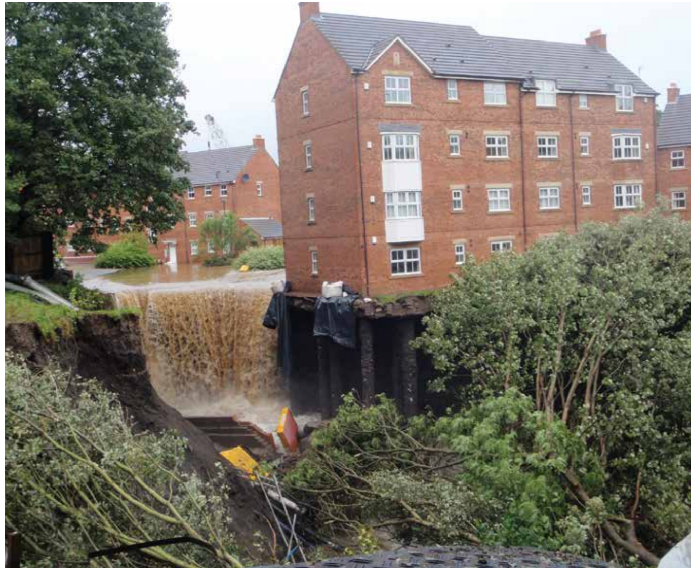
▲ Figure 3: Catastrophic damage caused by floods in north-east England in 2012. (© Tyne and Wear Fire Rescue Service)
