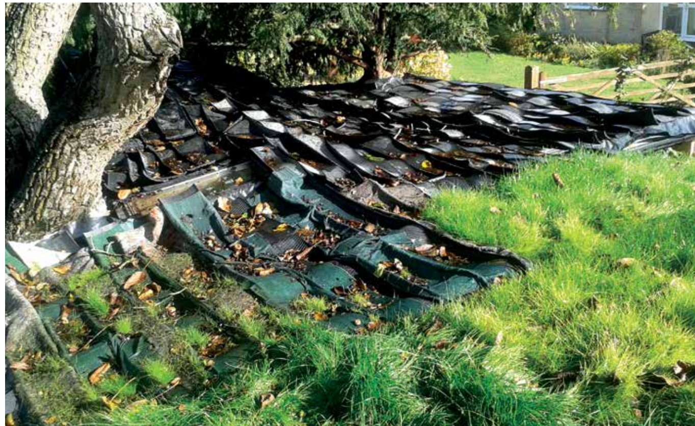
▲ Figure 1. Cut and arranged tyres forming the lattice roof of the Earthhouse (© Christopher Norris).
