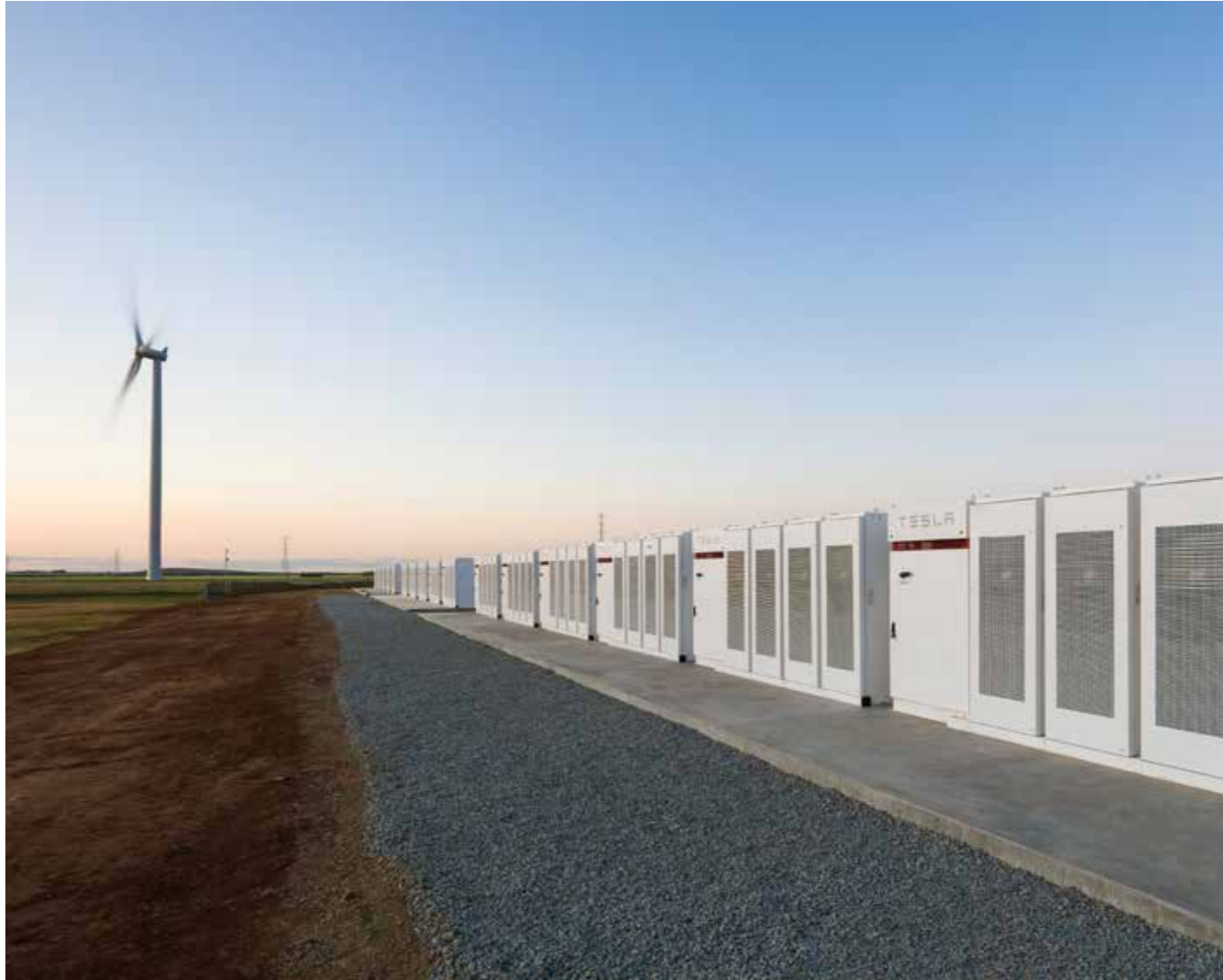
▲ Figure 1. In 2018, South Australia commissioned Tesla to install a 130 MV lithium battery system, then the world's largest, to smooth out the renewable energy supply from its wind farms and solar roofs. (© Liam West/Lightly Salted)
