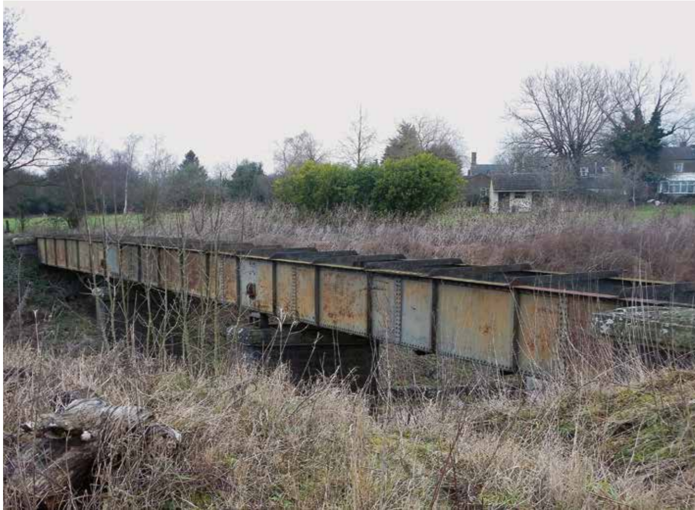
▲ Figure 1. This small, open-box aqueduct over the railway cutting carries the headwater of a significant river. It overtops regularly during high flows, which contributes to flooding in the cutting. (© Mark Everard)
