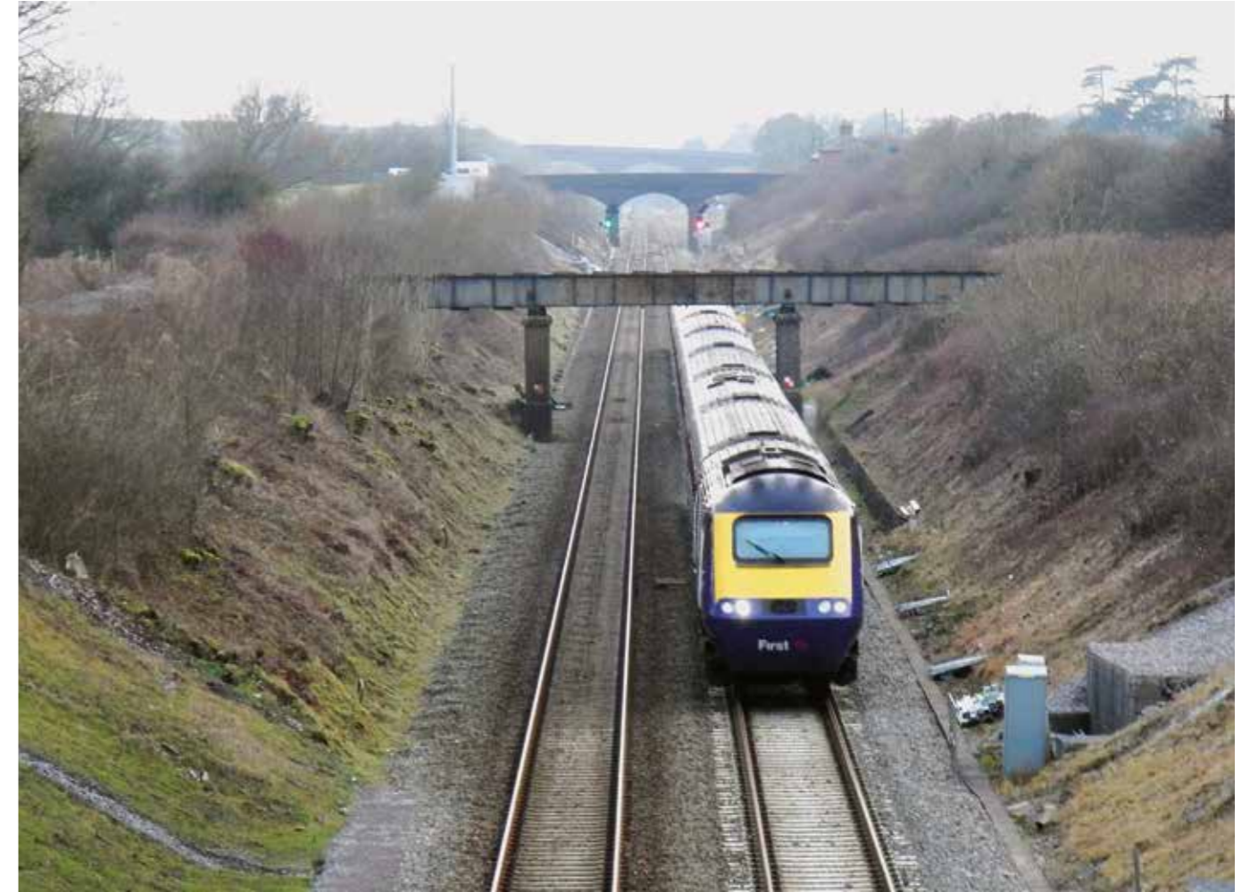
▲ Figure 2. On a major intercity route, a high-speed train passes under the open-box aqueduct in the railway cutting. Groundwater and surface flooding of the cutting frequently disrupt services at substantial cost. (© Mark Everard)
