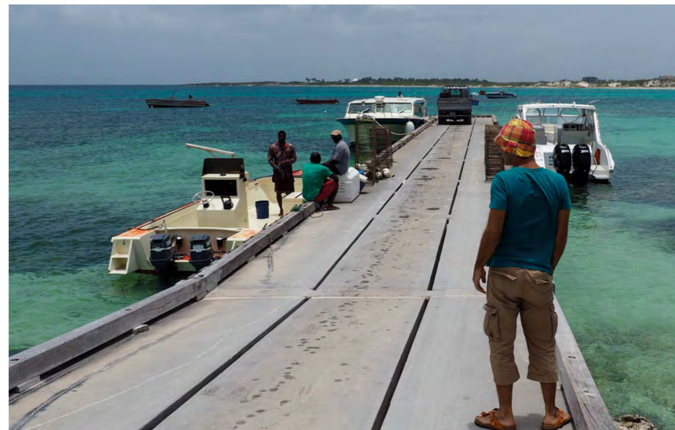
▲ Figure 2. Anguilla in the Caribbean – a typical low-lying community vulnerable to storm surges and tsunamis. The jetty is a robust structure potentially suitable for mounting sensors such as a tide gauge for storm-surge and tsunami warnings. (© Steve Hall)
