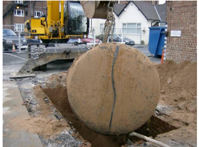
Figure 17: Empty tank being lifted
