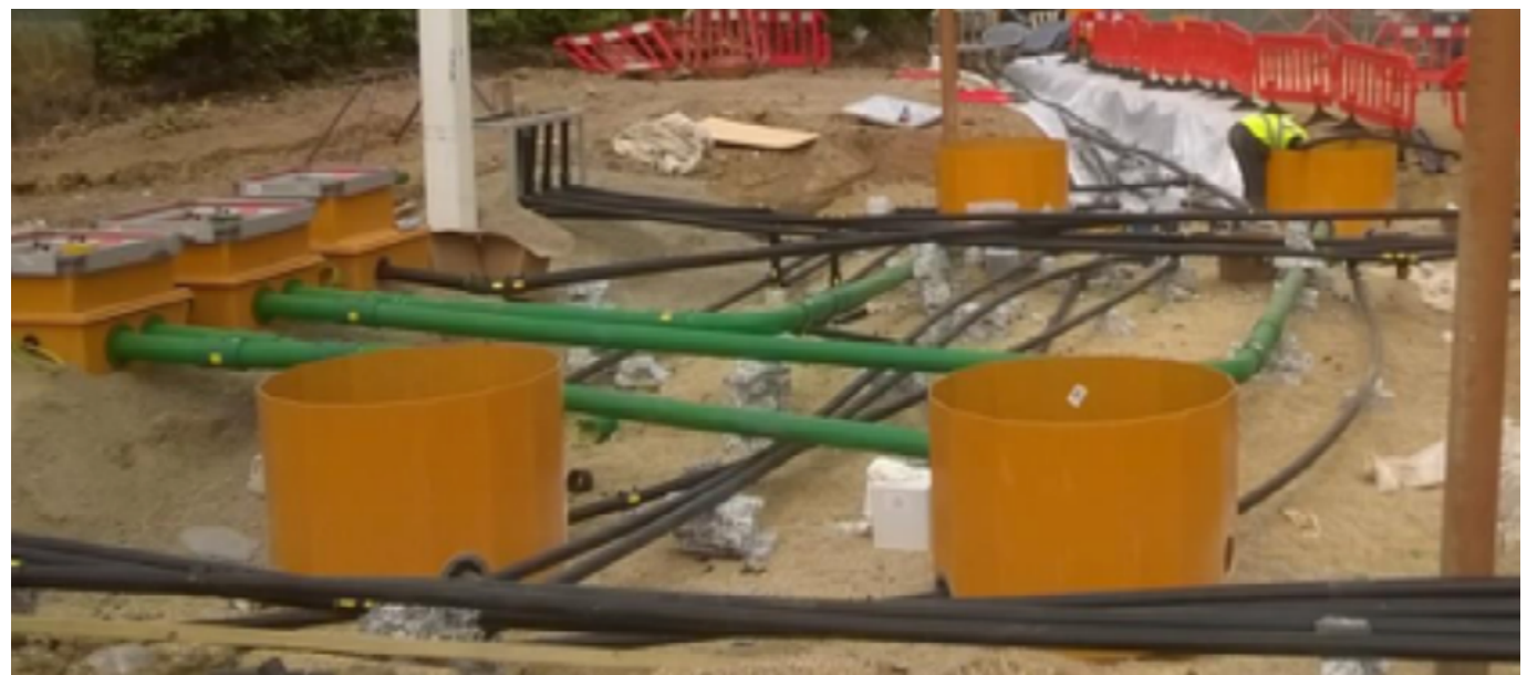
Figure 5: Typical modern forecourt in construction
