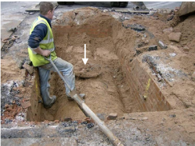
Figure 16: Identification of the pipe lifting point
