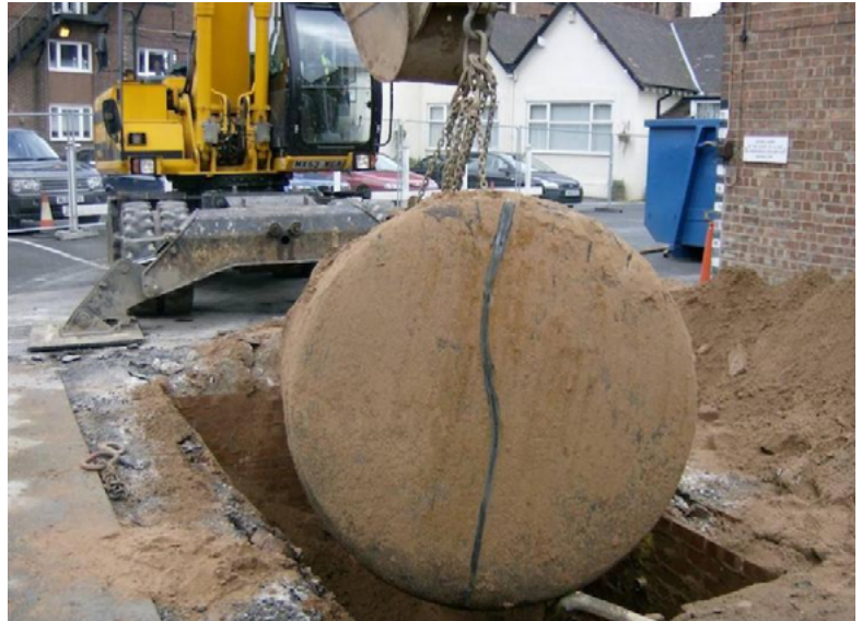
Figure 7: Removal of an underground tank
