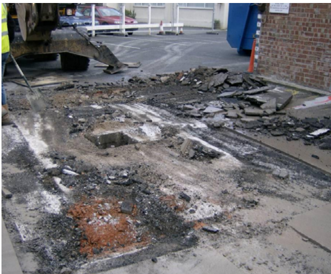
Figure 9: Top skin removed and area prepared for excavator with breaker
