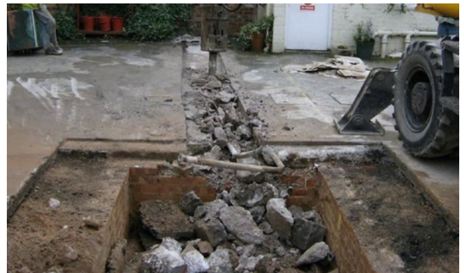
Figure 18: Pipework is removed and tank housing area is backfilled
