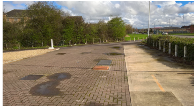
Figure 11: Inspection chambers at disused forecourt
