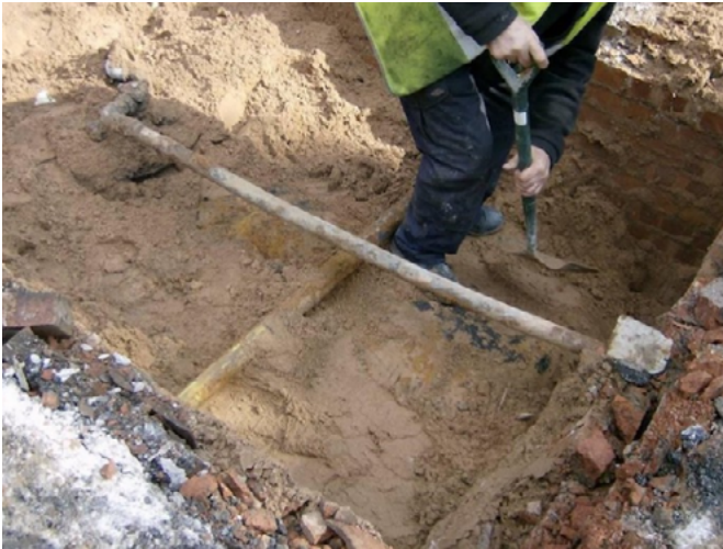
Figure 15: Bedding material being removed by hand
