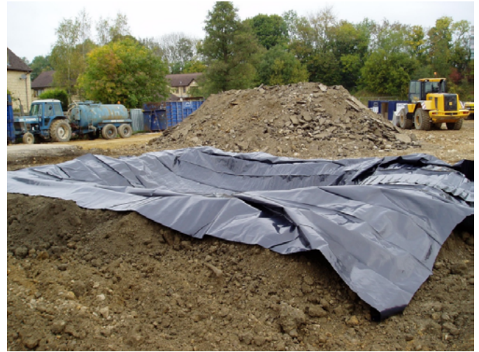
Figure 8: Temporary contaminated groundwater lagoon
