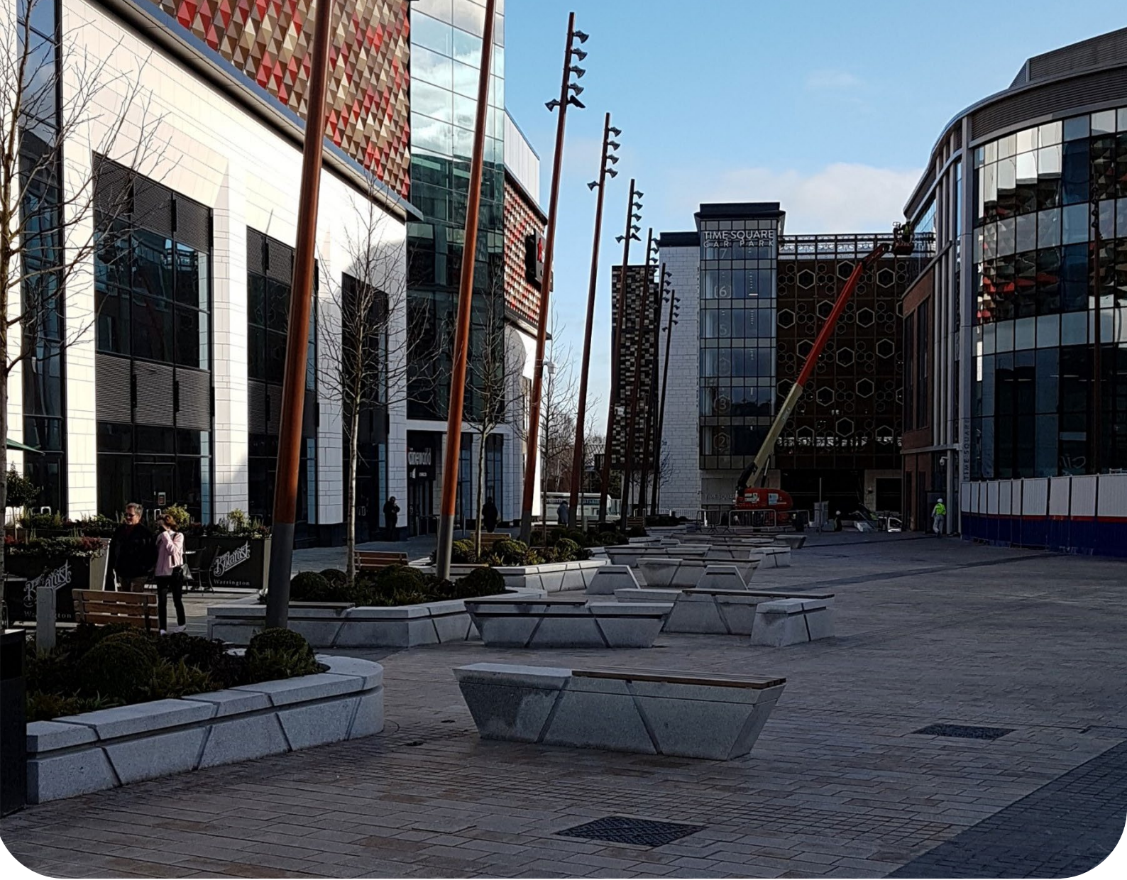
▲ Bridge Street Quarter: Cinema, council offices, indoor market and multi-storey car park on remediated gas works. Warrington, Cheshire. © Warrington Borough Council
