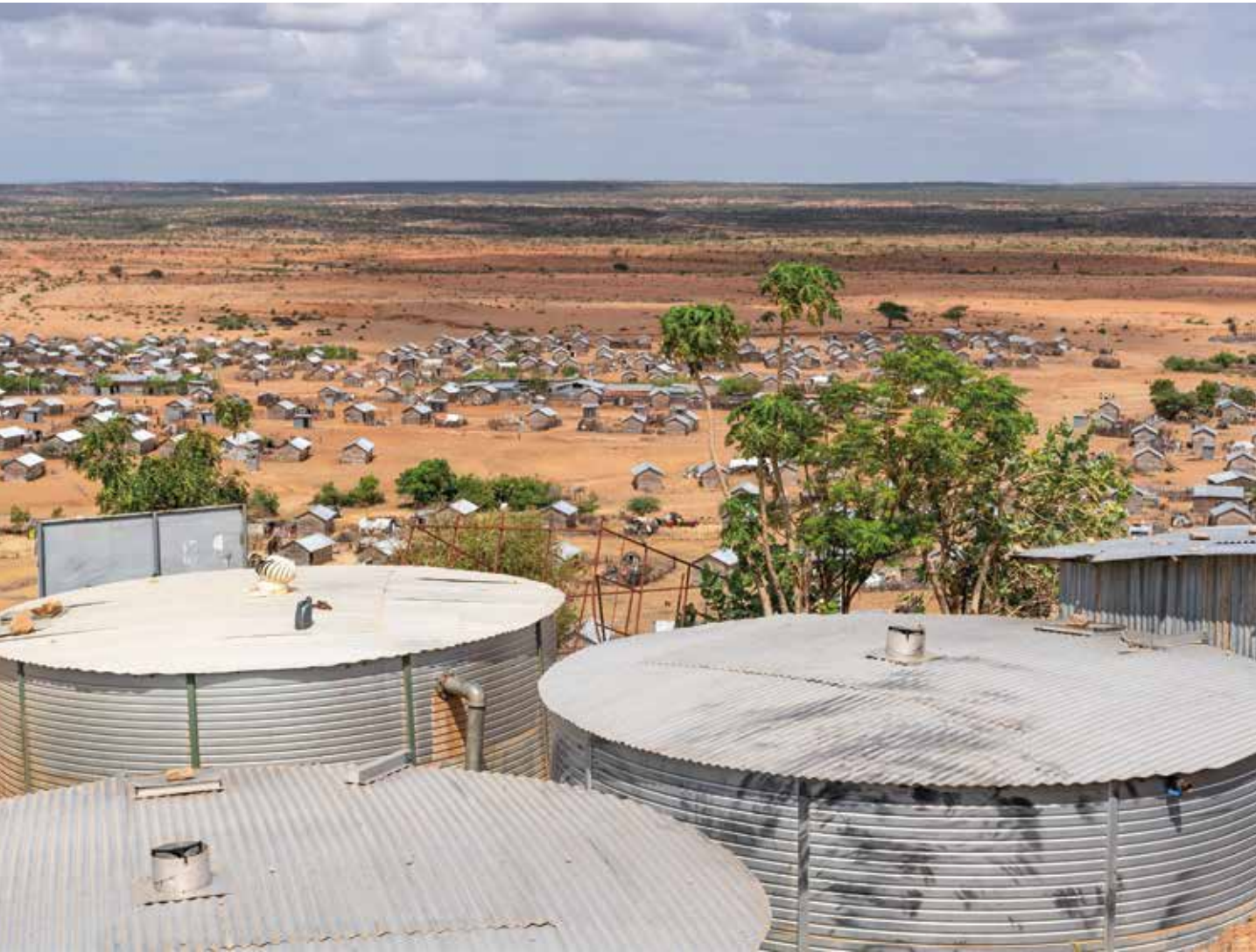
▲ Water supply tanks at Melkadida refugee camp, Dollo Aldo, Somali region. © Stanley Dullea | Adobe Stock
