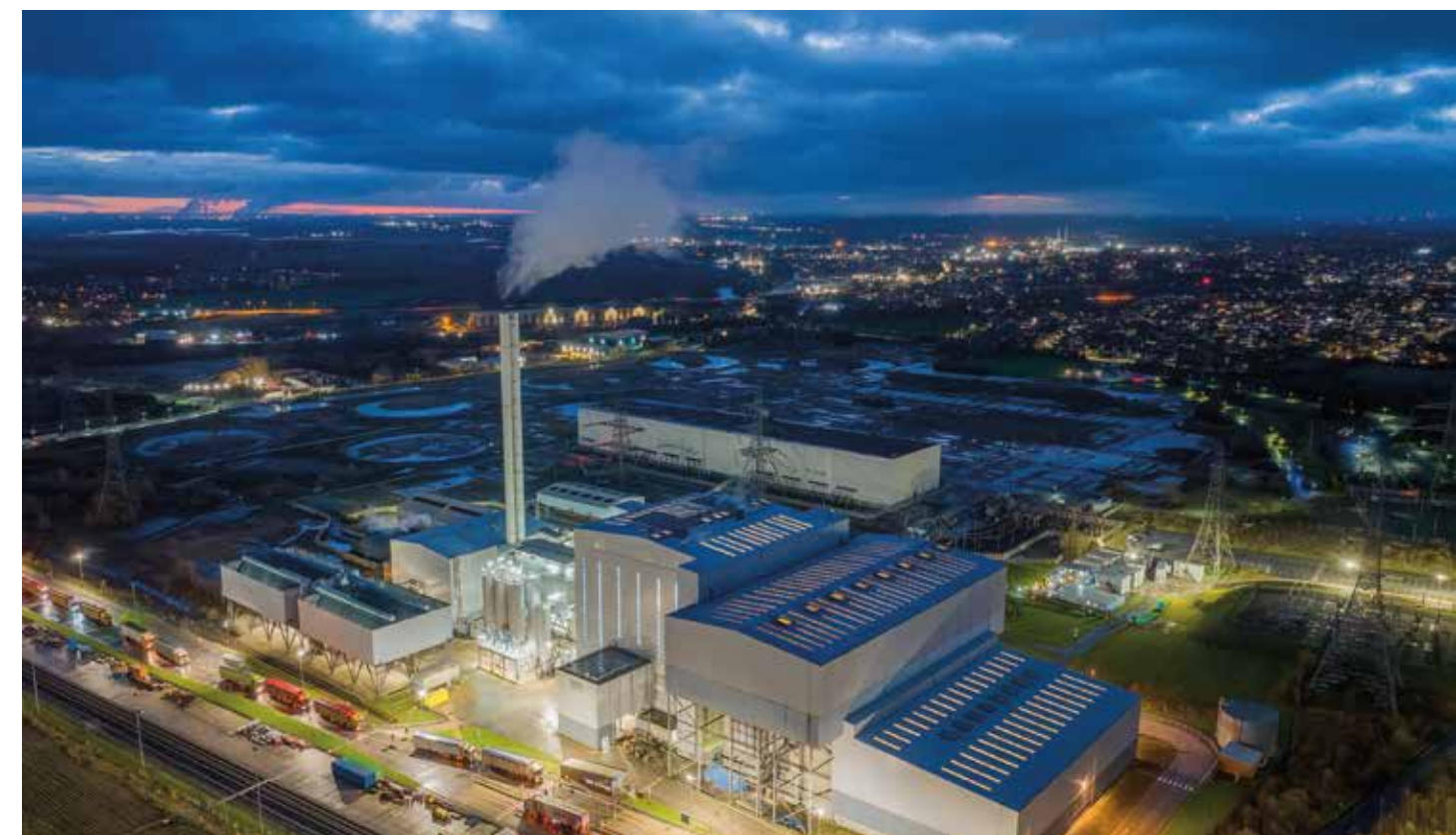
▲ Pilot carbon capture facility at Ferrybridge gas and multi-fuel power station, Yorkshire. © Chris Chambers | Adobe Stock
